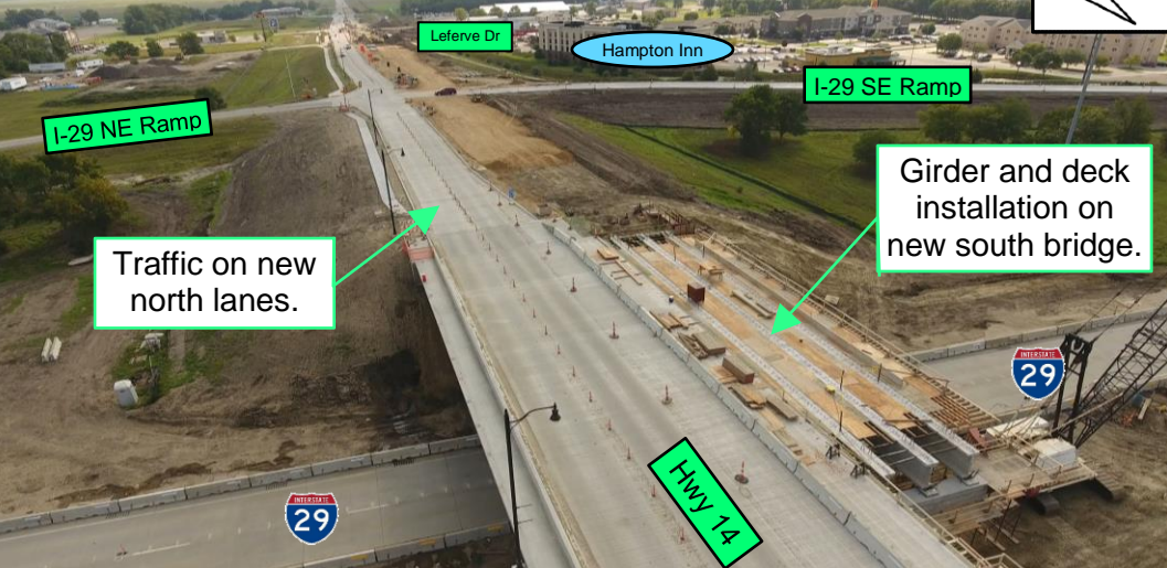
Project Photo: Work on the south bridge @ Hwy 14 (looking east)
